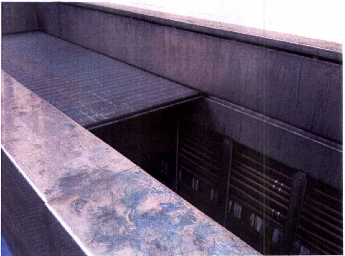
Degreasing plant with automatic shutters opening.
